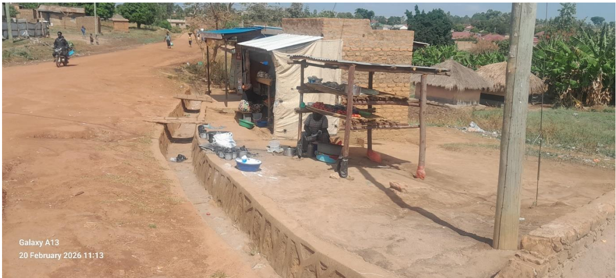
Figure 5. 8 Structures Along Alli Kenyi Road in Kiboko.
