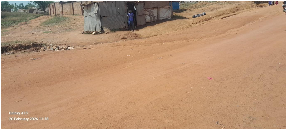
Figure 5. 6 Structures along Samuel Baba Road in Koboko TC
