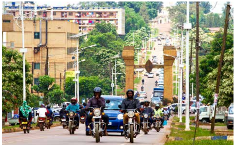
A well designed KCCA Road; Kabaka Anjagala Road Rubaga Division Kampala.
