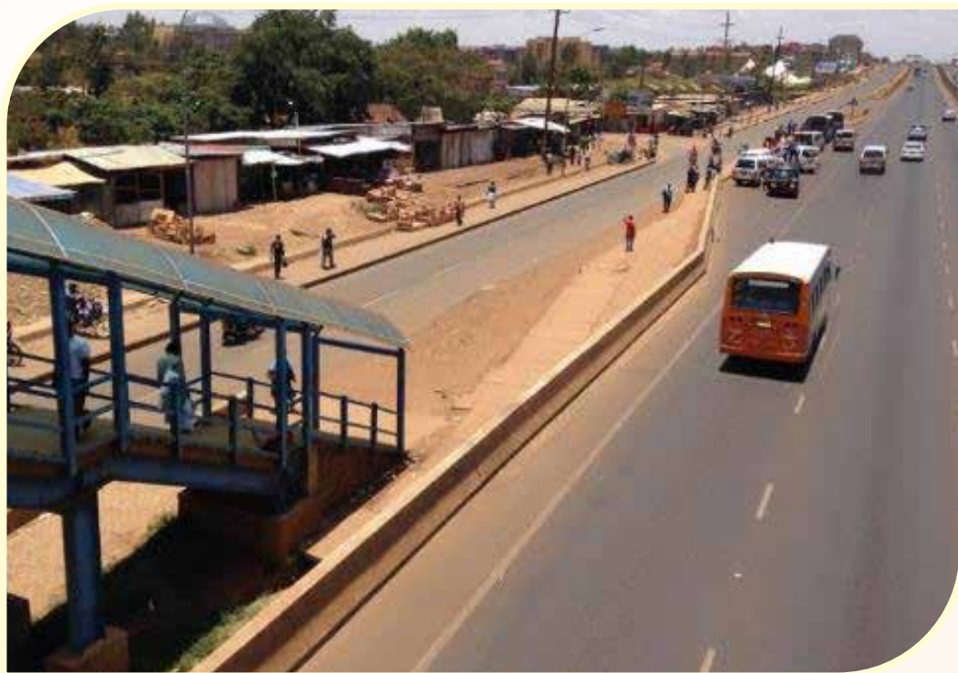
Figure 8-1: Example of NMT-vehicle separation at a public transport interchange
