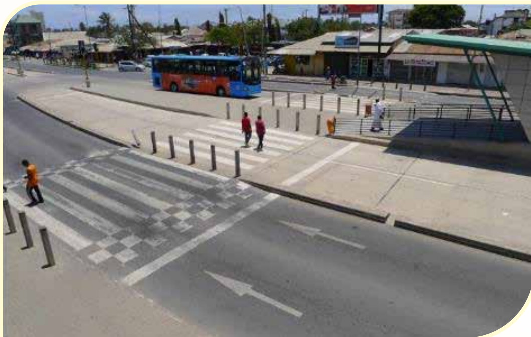
Figure 8-10: Photograph showing NMT access at a median public transport station
