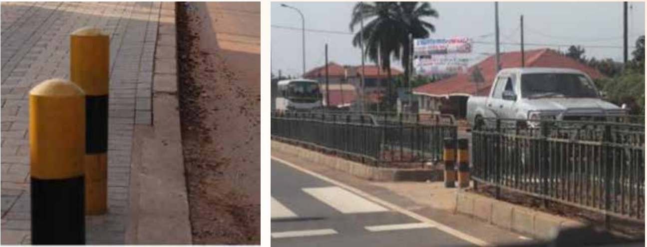
Figure 10-22: Dropped kerb with bollard protection
