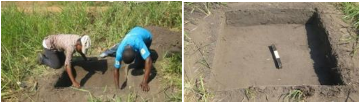
Plate 6-18: Test pit conducted in the road reserve
