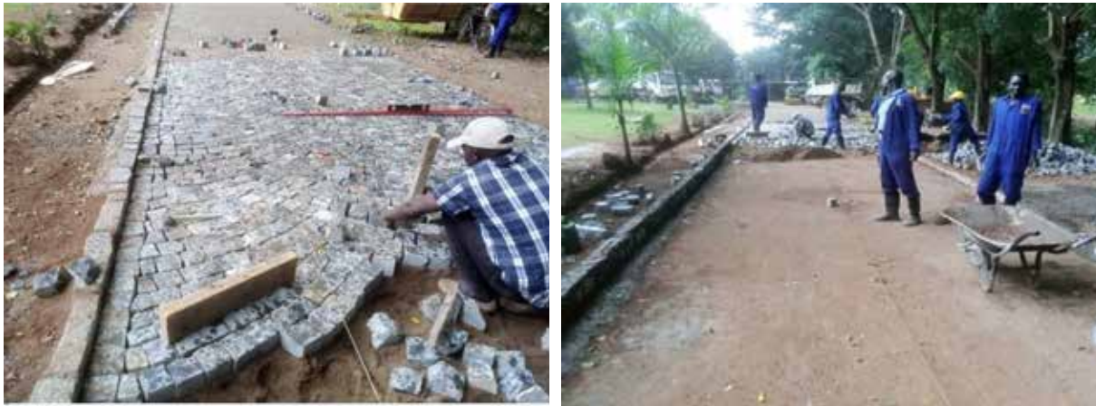
Laying of the cobblestone
