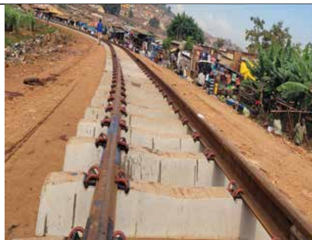
Laid sleepers on one of the sections
