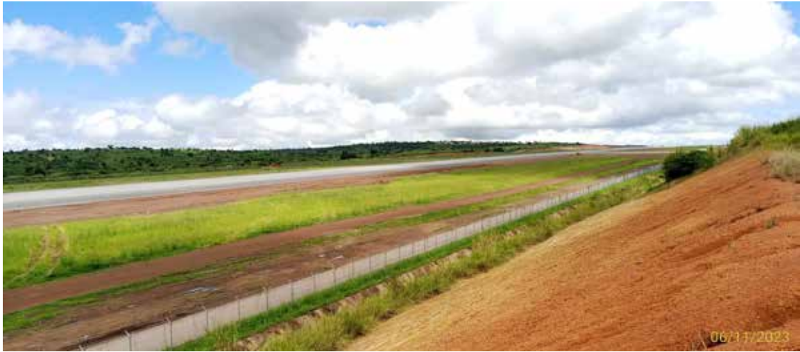
Kabaale International Airport runway
