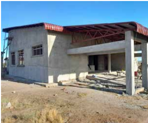
Fig (c) : New laboratory Block under construction at Moroto Regional laboratory
