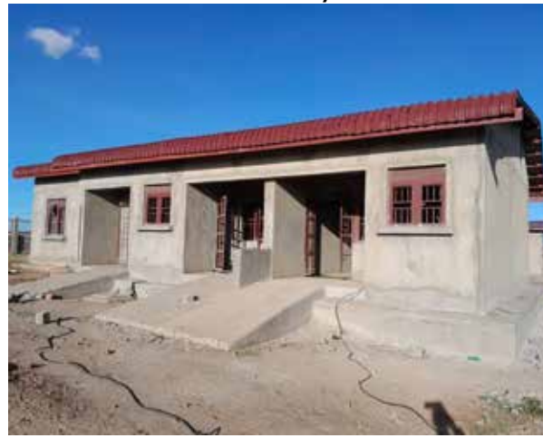
Fig (d): Staff quarters under construction at Moroto Regional Laboratory
