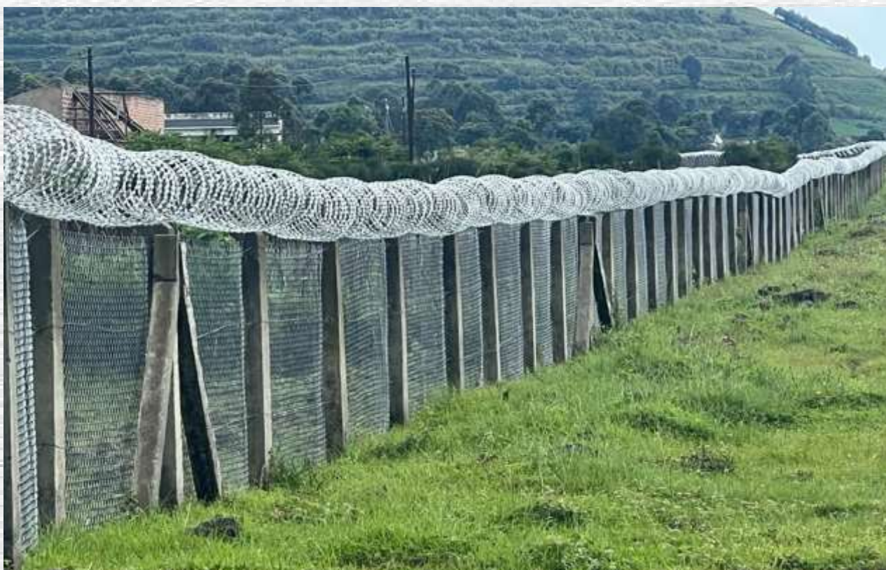
A Section of Kisoro Aerodrome perimeter fence newly constructed.
