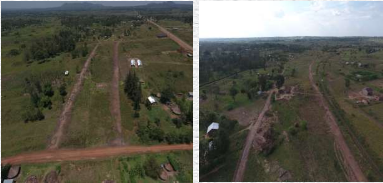
Aerial view of cleared and demarcated SGR ROW in Tororo District
