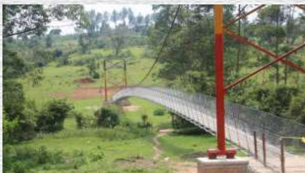
Kasumbelya Trail Bridge
