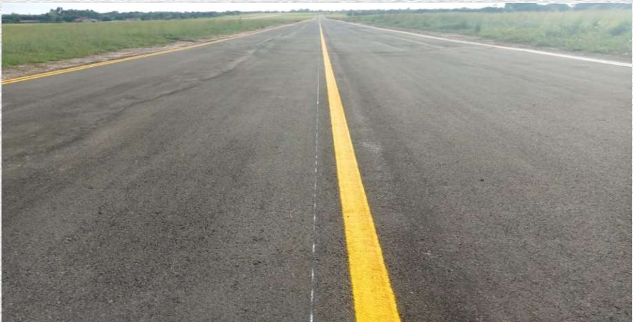
Construction of A Taxiway Link at Soroti Airport 100% complete
