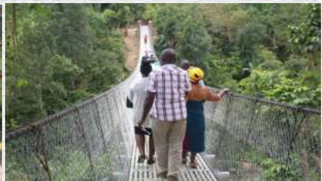
Masaka - Munsiso Trail Bridge
